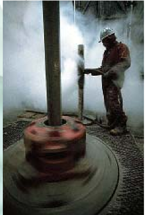
Drilling for Oil in the NWT
