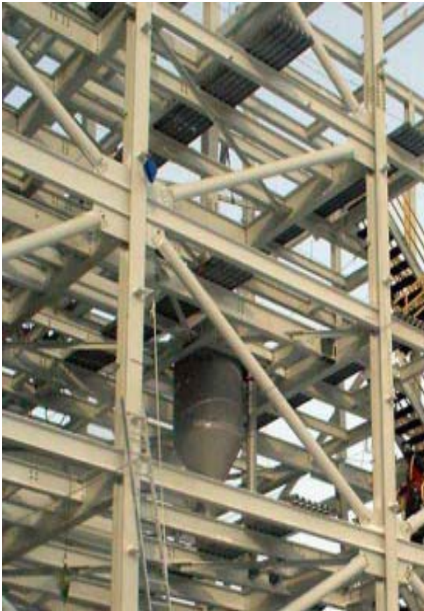
Construction at Diavik Mine
