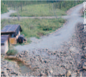
The pump house at Colomac Mine removes excess surface water.
