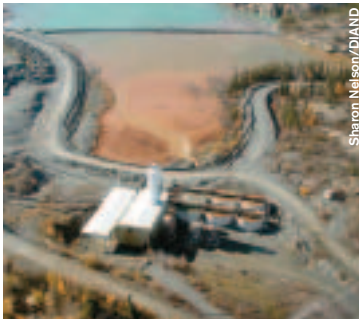
The settling pond sits behind the Effluent Treatment Plant. (Giant Mine.)
