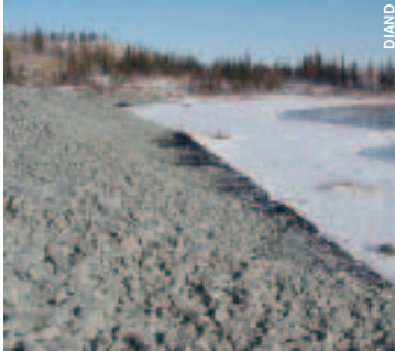
Potentially contaminated water is contained at the mine site. (Giant Mine.)
