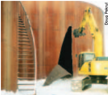
Remediation at Colomac Mine.
