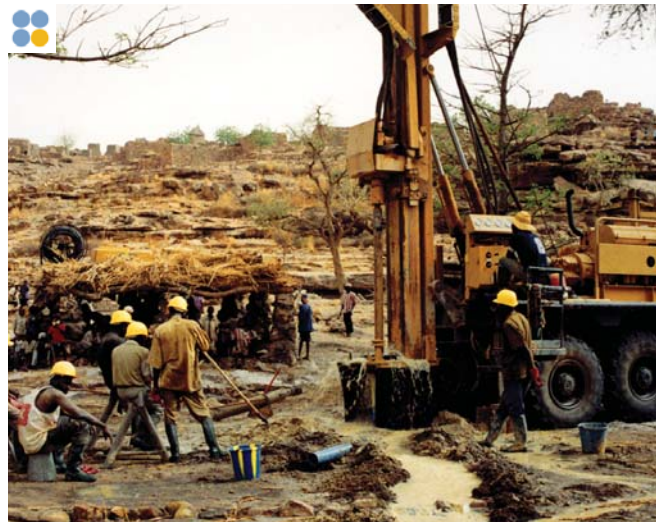
photo: TECSULT (Groundwater Drilling-Mali)
