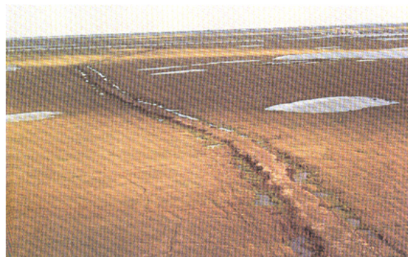
FIGURE 6.2-2 FLOW SLIDE ALONG DEMPSTER HIGHWAY CAUSED BY CUT INTO ICE RICH SOIL AND WATER ACCUMULATION AND SLUMPING ALONG A ROAD BUILT IN PRUDHOE BAY
