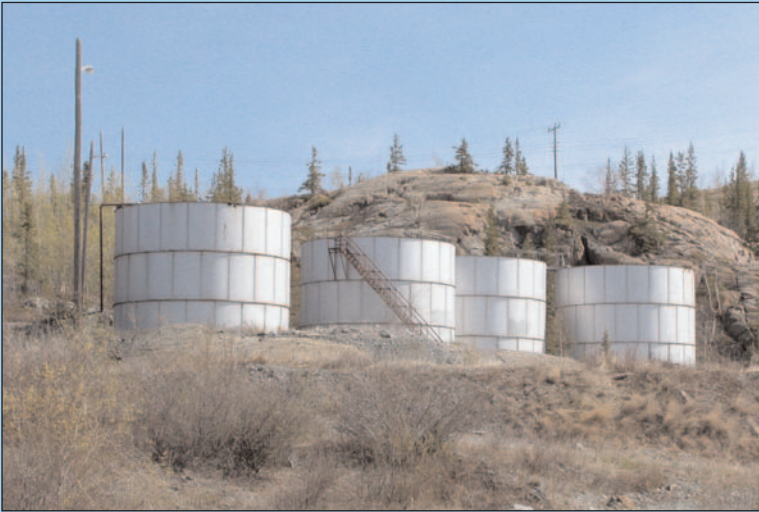
Fuel storage tanks before demolition.
