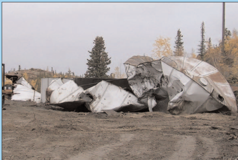
Taking down the tanks.
