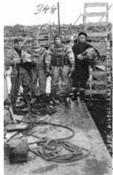
Figure 2.72 Divers Building the Dam at Rapides-des-Joachims
