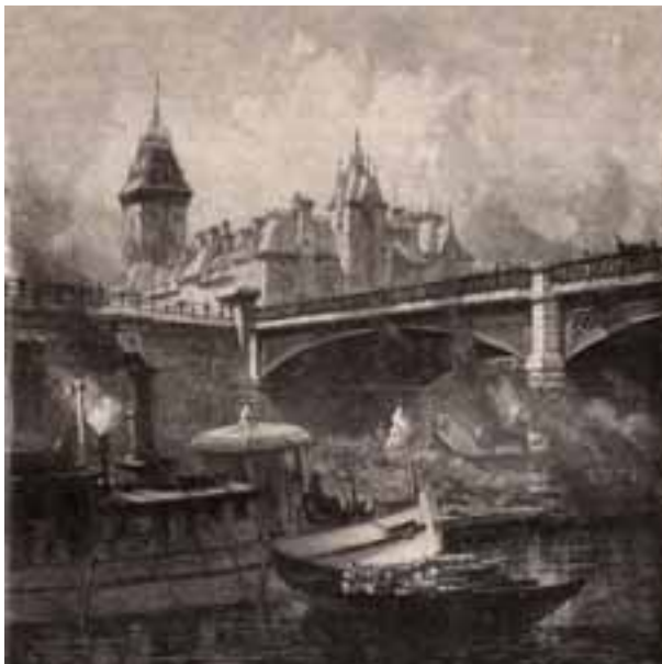
Figure 2.36 Under Dufferin Bridge
