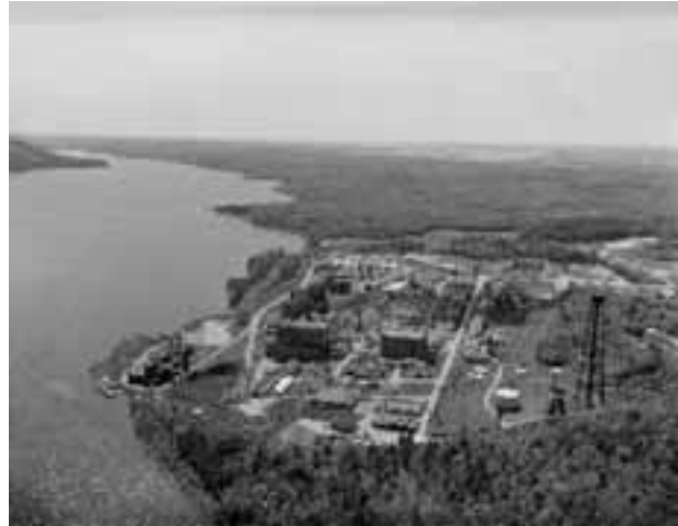
Figure 2.78 Pointe au Baptême Showing the Nuclear Power Plant
