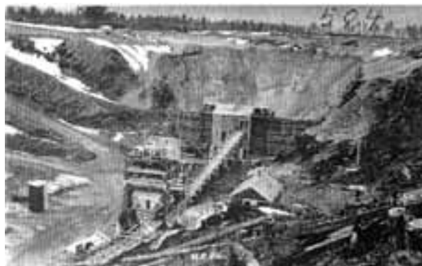
Figure 2.77 Building the Dam at Rapides-des-Joachims
