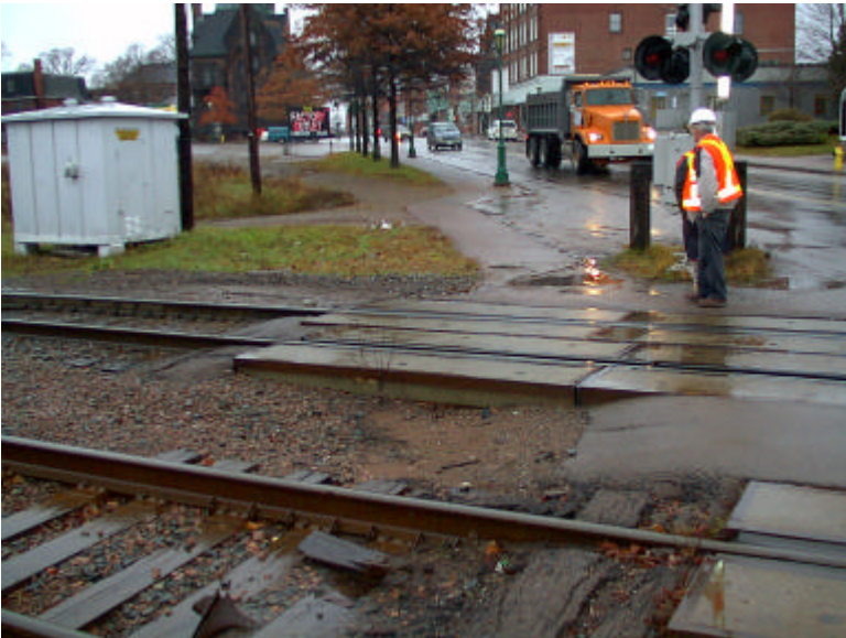
Photo 5: non-contiguous crosswalk on west side of crossing
