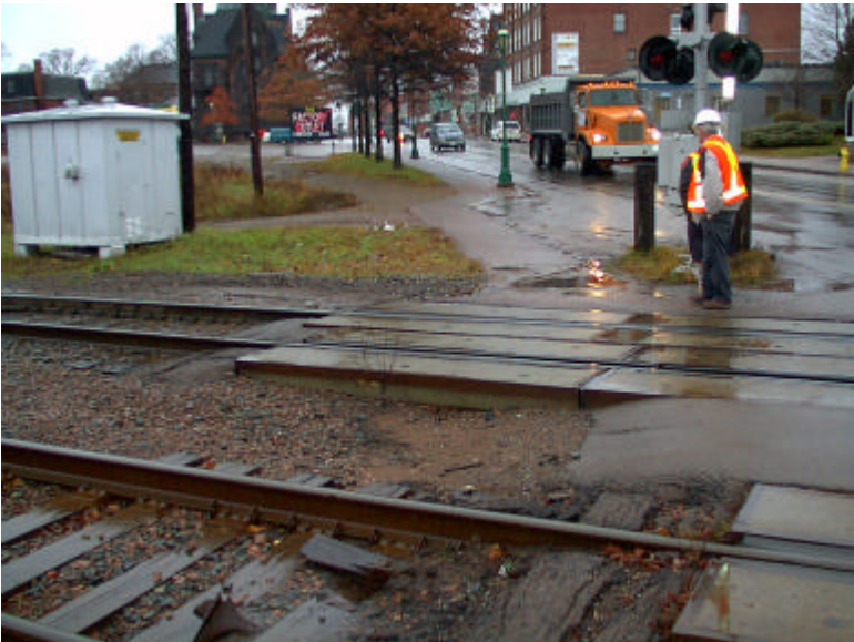
Photo 5: non-contiguous crosswalk on west side of crossing
