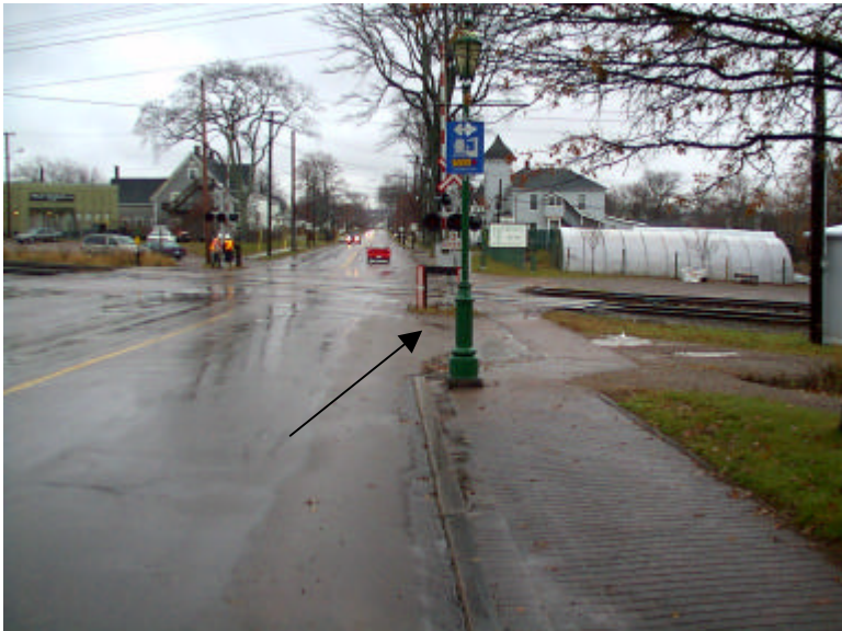
Photo 3: Southbound Main showing alignment of gate hardware
