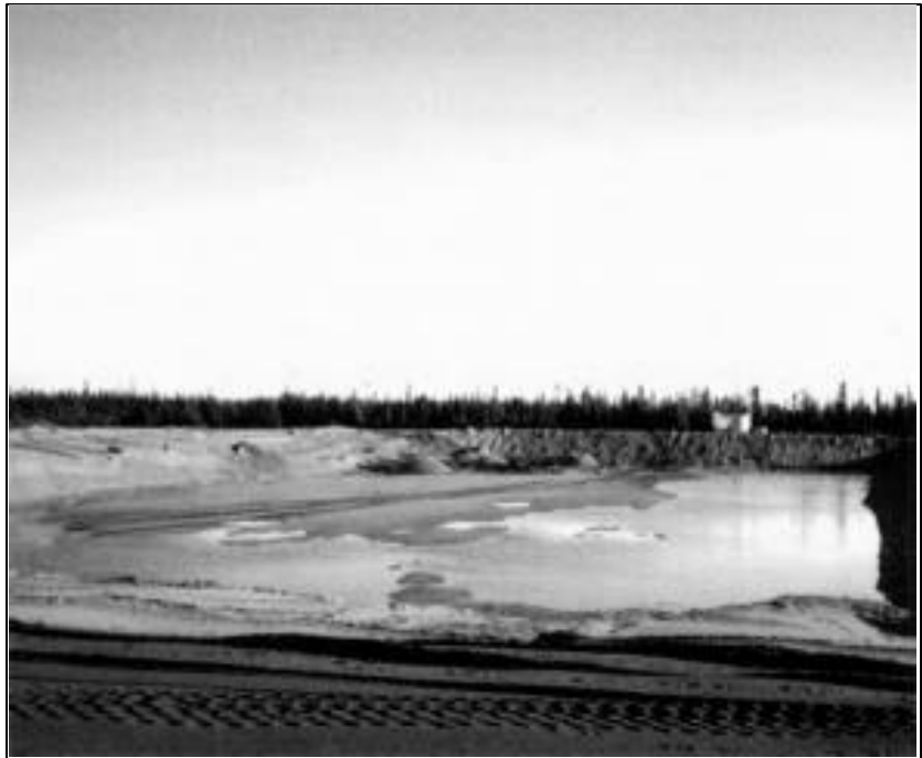
Construction of a new sewage system in Chisasibi.
