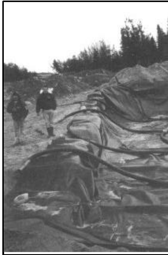
In 1998, a biotreatment pad for soil decontamination was installed in Waswanipi.
