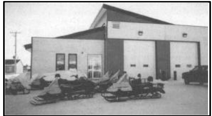
Outside view of the Whapmagoostui fire station.
