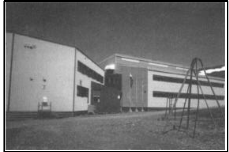
Kangiqsujuaq School. Because of the rock-hard ground, permanently frozen by permafrost, soil characteristics and rock, most Nunavik schools have to be built on pilinas.
