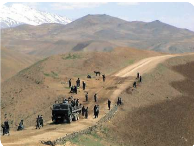
Road Repair, Hazarajat
