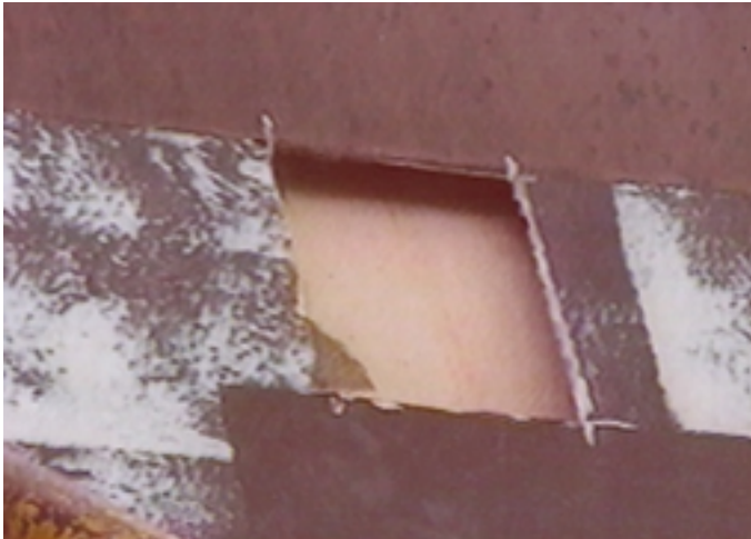
Missing insulation.
