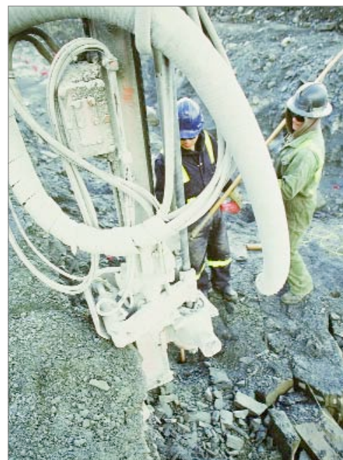
Work being done on the barrier wall
