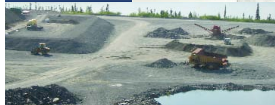
Overview of the Land Treatment Unit (LTU)
