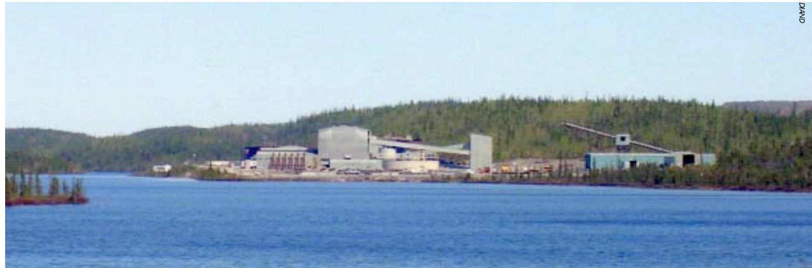
A view of the millsite at Colomac
