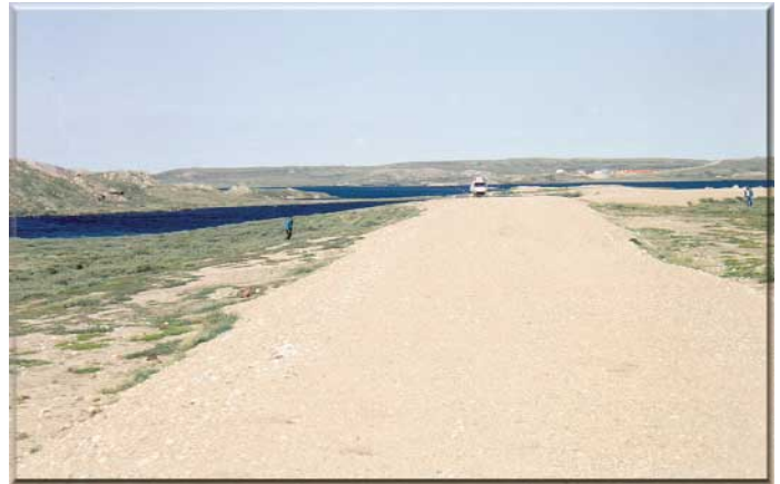
Photo 5. Winter road portage (Site 3), Echo Bay road camp in background.
