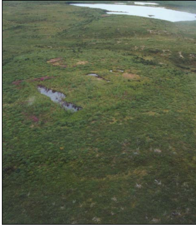
Figure 7a. Subsidence and ponding on sump cap, (Gulf Mobil Siku C-11) Parsons Lake area. The standing water has accumulated due to subsidence of the sump cap. Photograph: Summer 2000.
