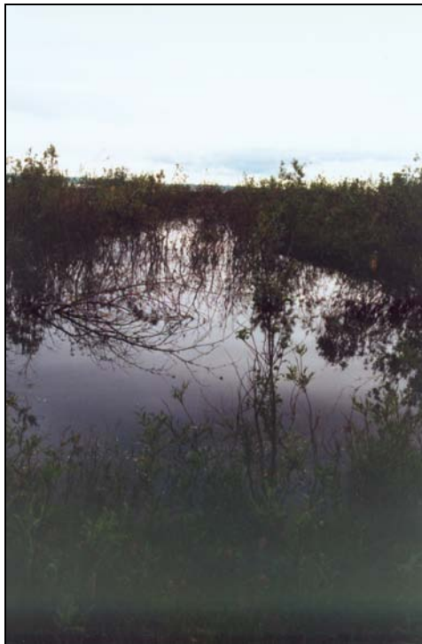
Figure 7a. Subsidence and ponding on sump cap, (Gulf Mobil Siku C-11) Parsons Lake area. The standing water has accumulated due to subsidence of the sump cap. Photograph: Summer 2000.
