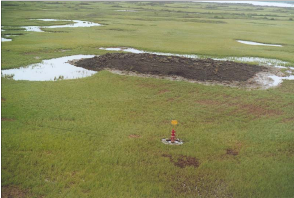
Figure 13. Ponding of water around recently constructed sump (Kirk M-15), Mackenzie Delta.
