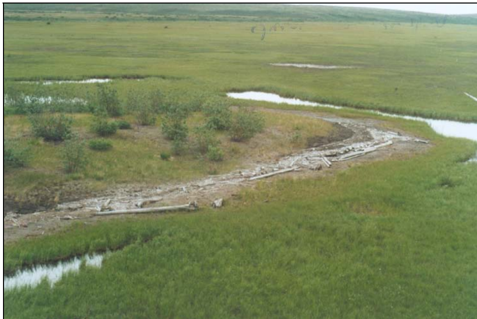
Figure 8. An intact sump (Gulf Mobil Ogeoqueoq J-06) in the Parsons Lake area. Note that the sump cap is largely unvegetated and that the site is well-drained. Photograph: Summer 2000.
