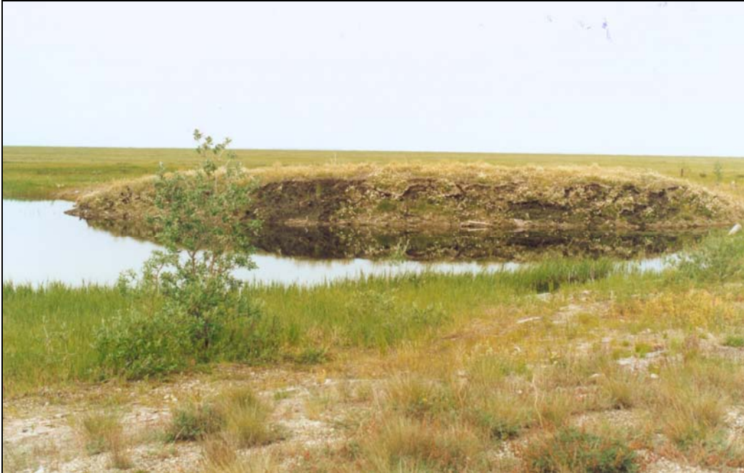
Figure 11a. Sump cap collapsing into an adjacent thaw pond in the Taglu Island area, Mackenzie Delta. Photograph: Summer 2001.
