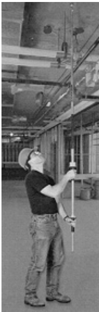
Extendable arm for power and impact tools (patent)
