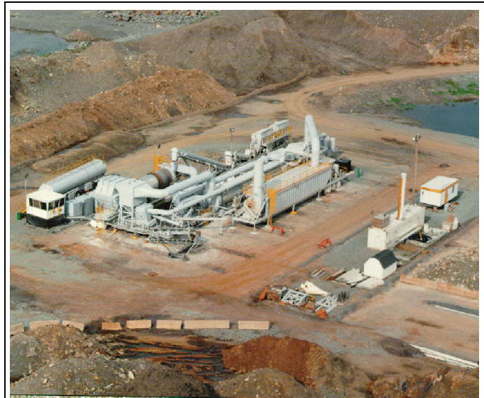
Figure 5.3 Thermal Phase Desorption Unit
