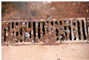
Lack of proper containment during antifouling paint removal can result in deleterious substances being released into the aquatic environment.
