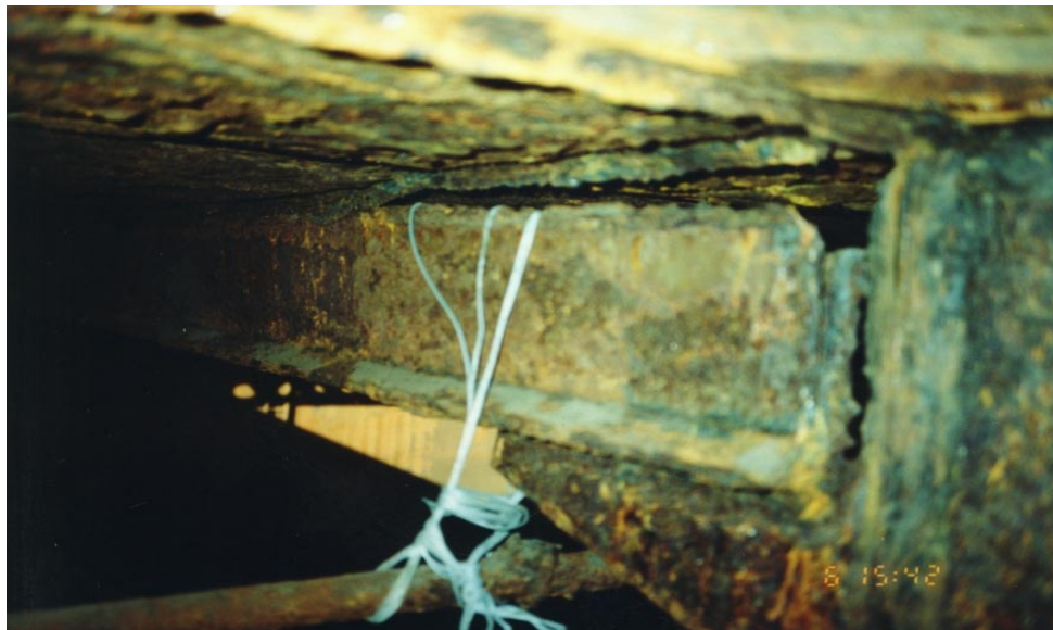
Severe corrosion of underdeck structure on a bulk carrier
