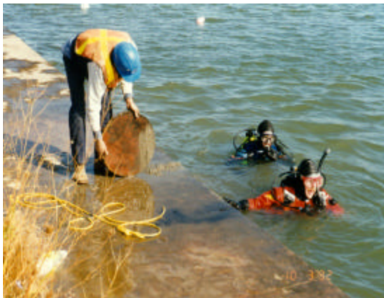
Divers removing debris manually from the demonstration area
