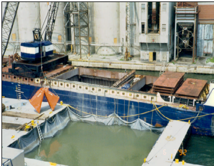
View of working cell and holding barge
