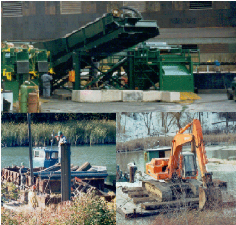
View of treatment plant and sheetpiling and backfilling operations
