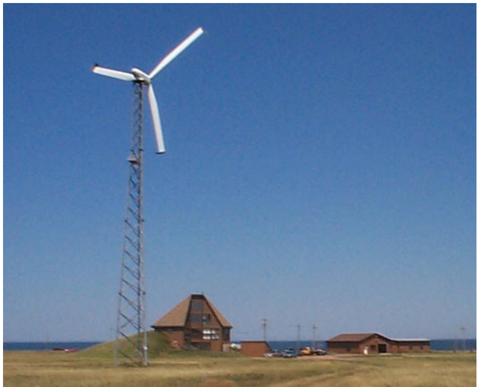
(Caption fig 2 Enertech 40 kW overlooks the main office and workshop.)
