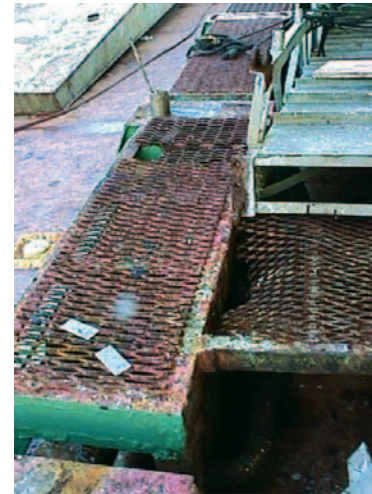
Corroded gratings
