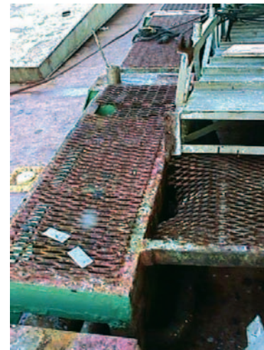
Corroded gratings
