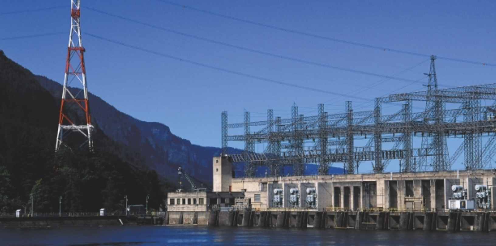
figure 2: Powerhouse at Hydroelectric Dam
