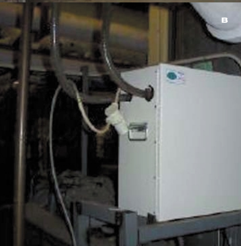
figures 19A & 19B: Amalgam Separators at The Hospital for Sick Children SOURCE: The Hospital for Sick Children
