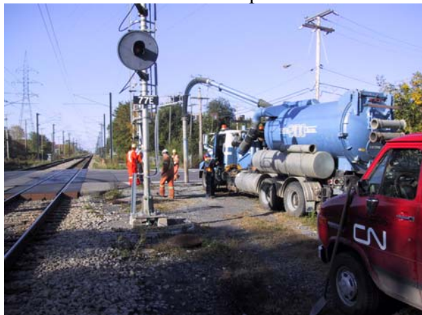
Installation des poteaux
