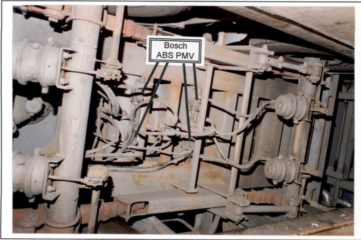
c) Pressure Modulating Valve - PMV (4-Channel Pup Trailer Configuration)
