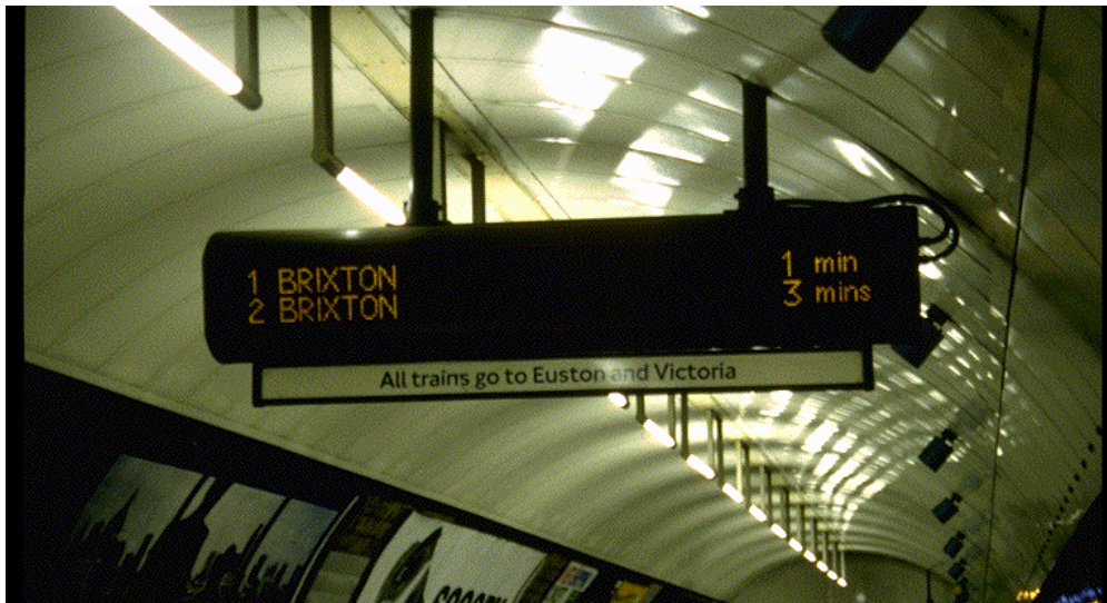
Figure 11 Displaying the waiting time and destination for the next few services. This display is in the London underground (subway). Similar displays are being introduced at bus stops in many European cities. In Southampton, a transponder carried by visually impaired people triggers audio announcements of the information displayed.
