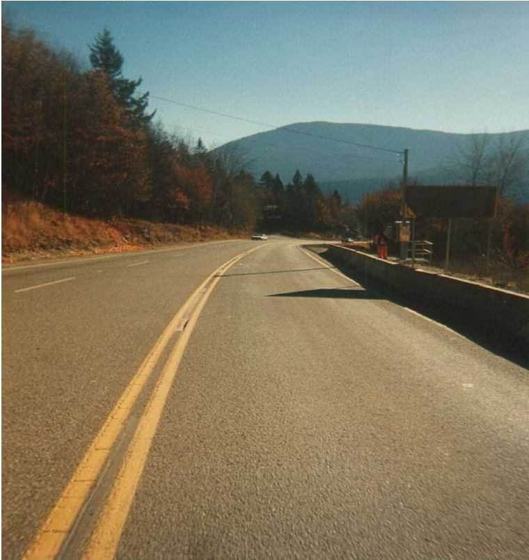
Figure 2-3 Road Segment with Sensors (located adjacent to the pole)
