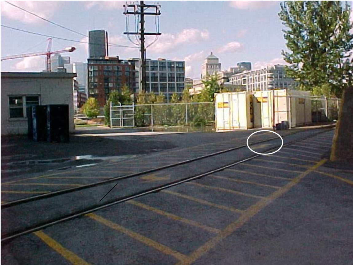
Figure 23 Location where the eastbound wheel sensor should have been installed
