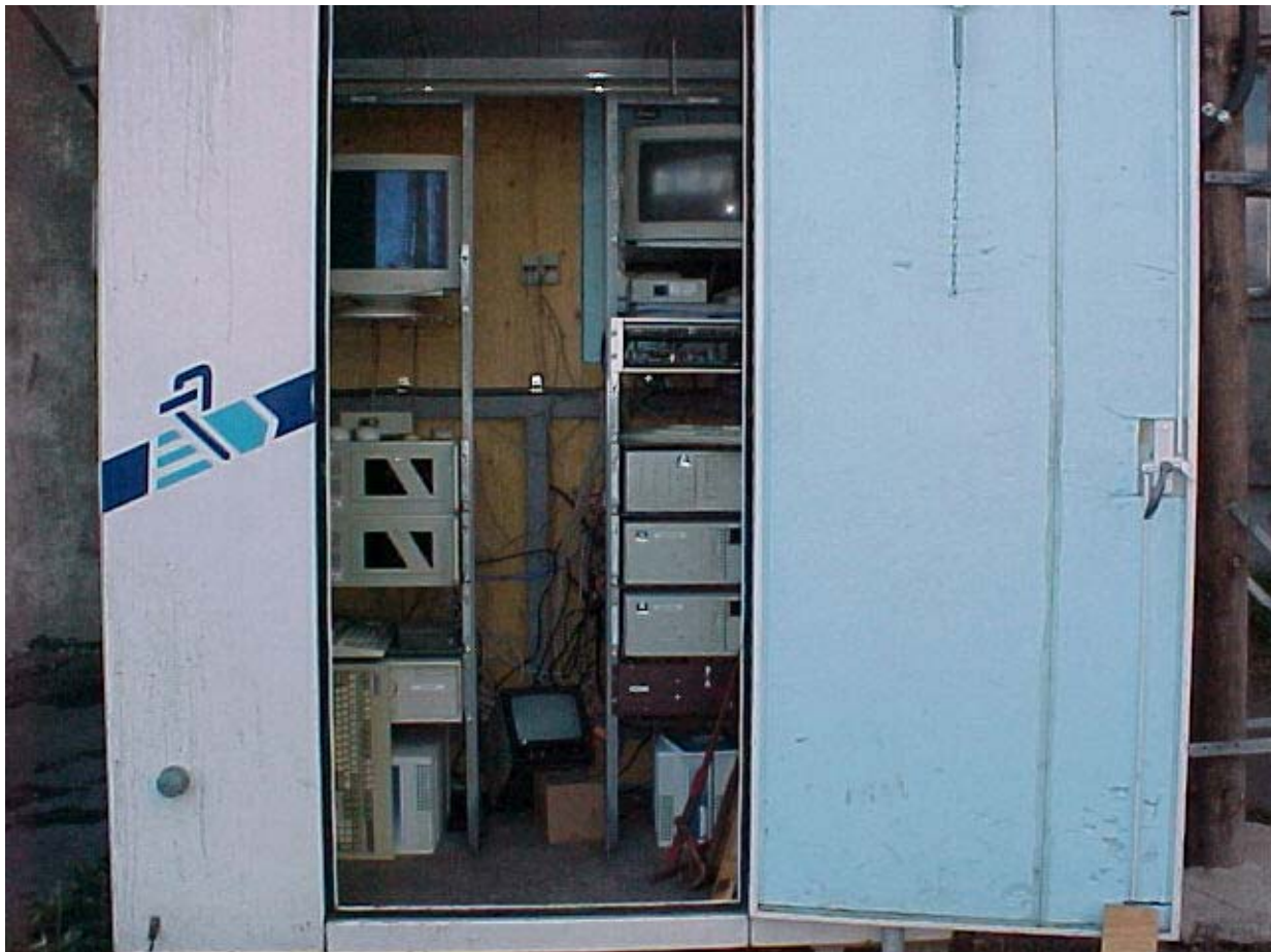
Figure 24 Bungalow – front view
