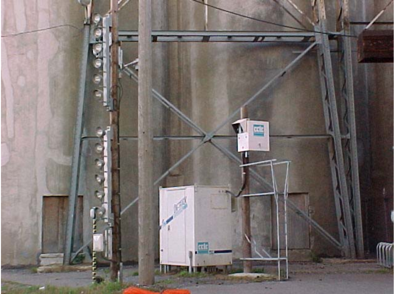
Figure 1 Picture of the site near elevator No. 5
