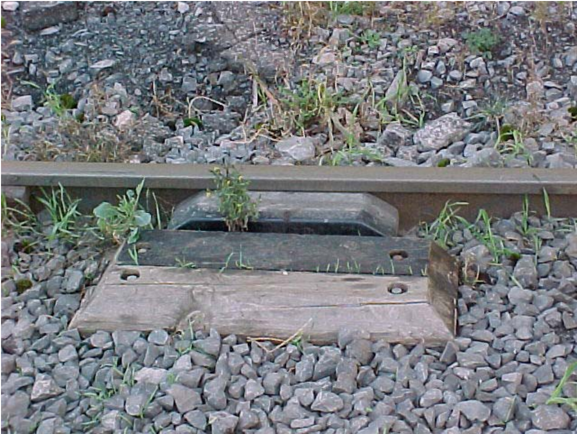
Figure 19 Close-up of the wheel sensor with protective bar
