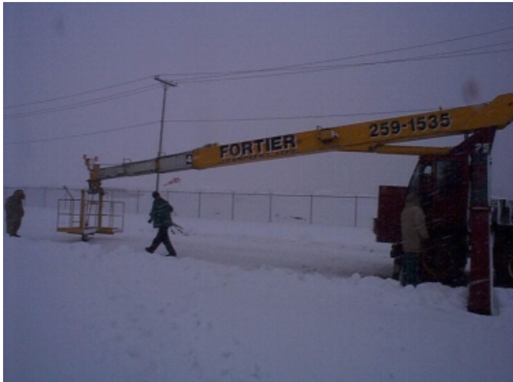
Photo 2.2: Personnel Basket Installed on Mast
