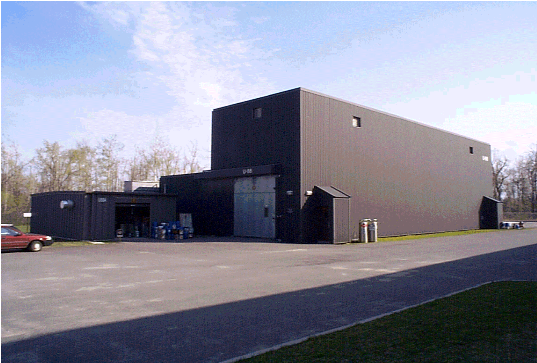
Photo 2.3: Outdoor View of NRC Facility
