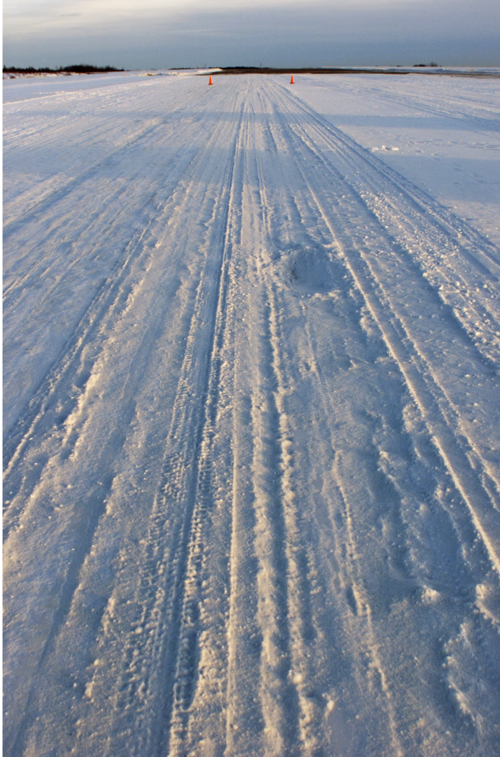
Figure 5b. A general view of the altered conditions of the compacted snow strip on the east side of runway 13-31 after all the ground vehicle tests of 30 January 2002
