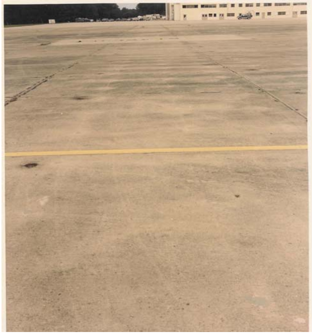
Figure K.1 Profiling site 1 on South side of Hanger N159
