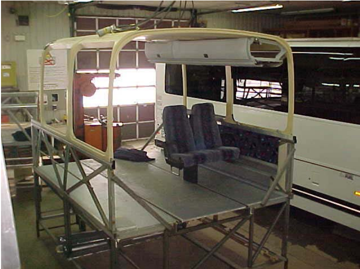
FIGURE 7: Mock-Up Installation of the One-Piece Composite Roof Module
