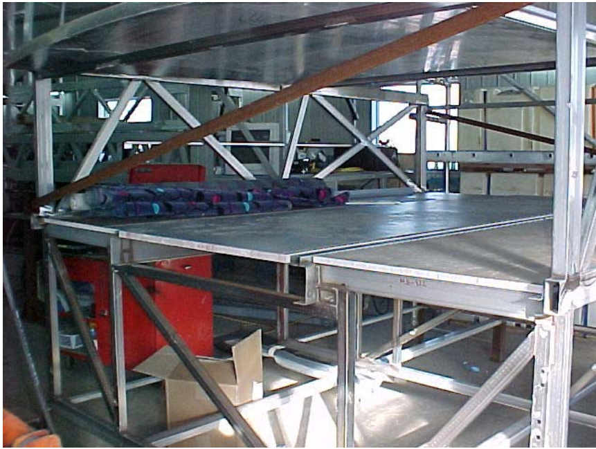
FIGURE 6: Mock-up Installation of Prototype Floor Panels
