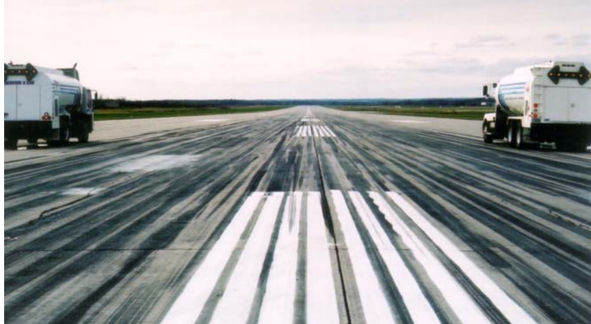
Figure 5 – Water Tankers Ready to Wet Runway 29 Test Section at Mirabel
