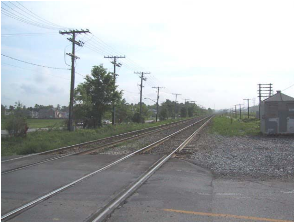
Woodland Avenue – Northbound Looking East
