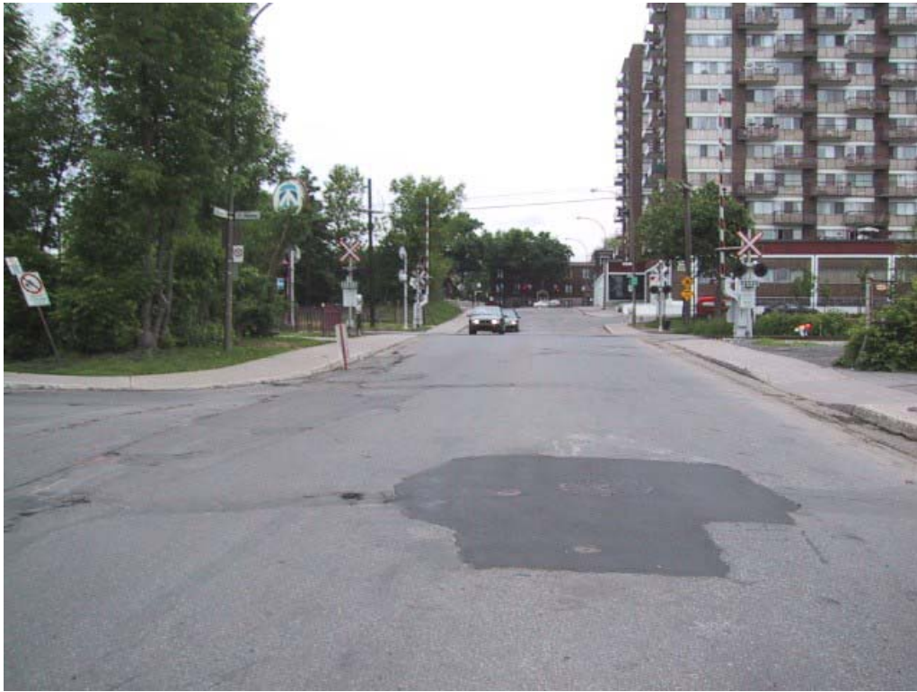
Elmhurst Street – Northbound
