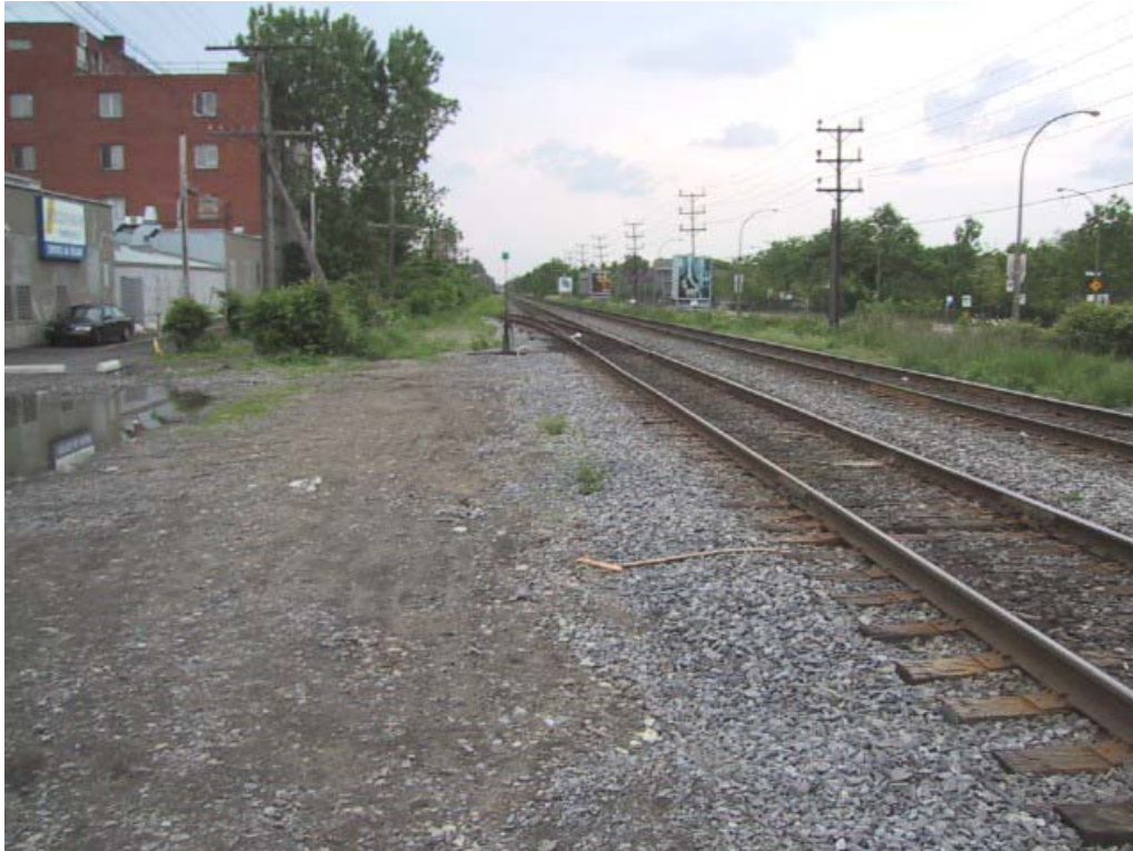
Wilderton Avenue – Northbound Looking West Along Tracks
