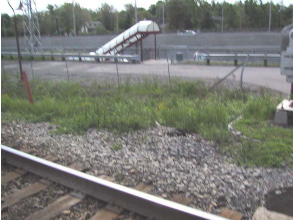
Baie d'Urfé – Pedestrian Tunnel to Street Level on South Side
