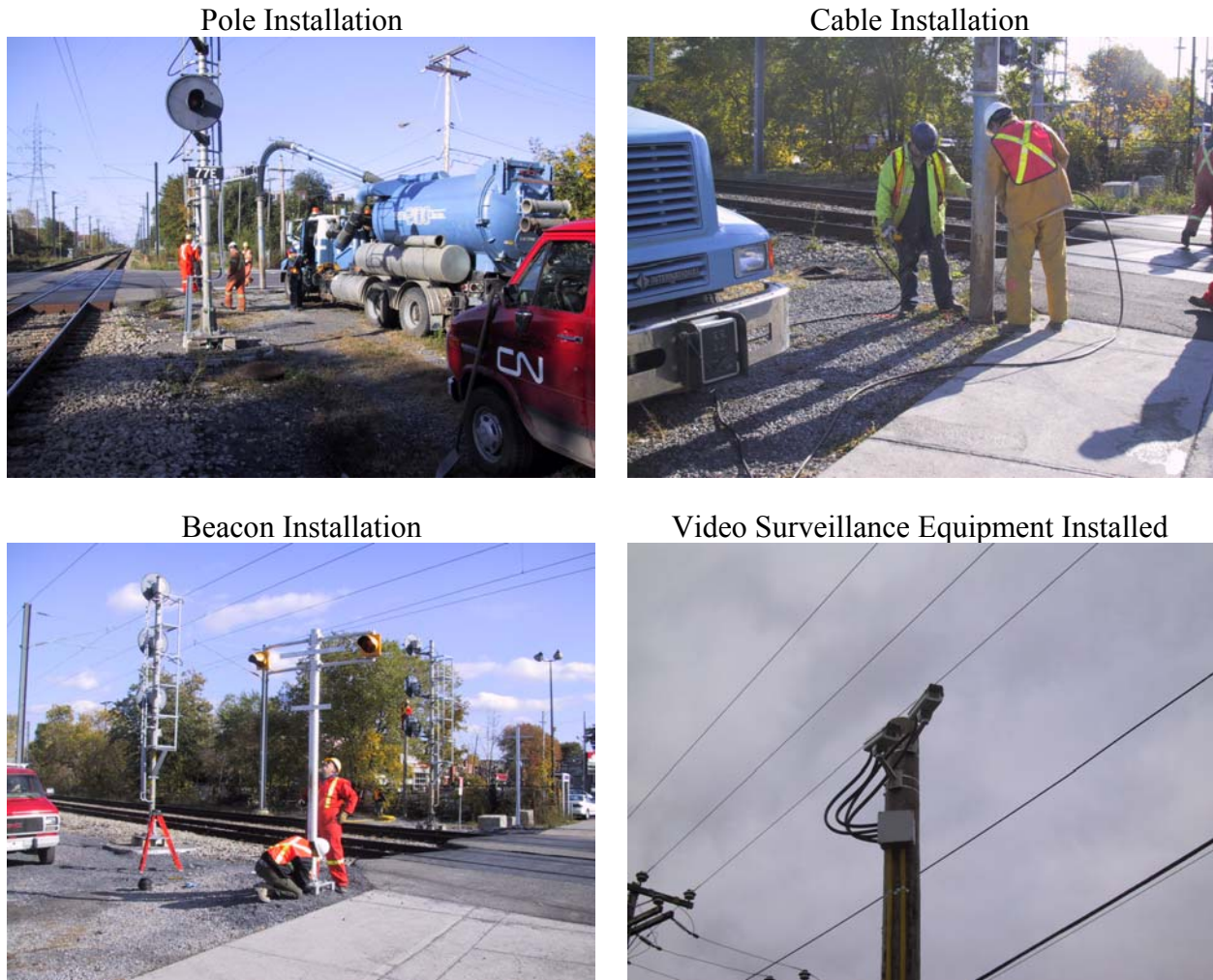
Figure 11-1 STW System Installation
