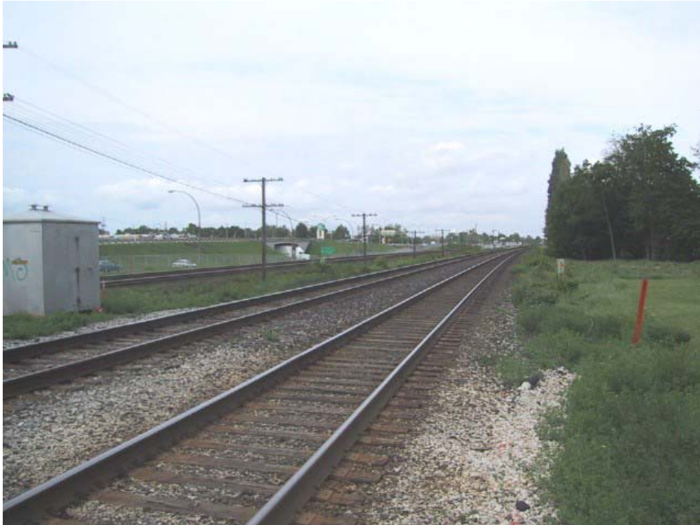
3 e Avenue – Southbound Looking West Along North Tracks
