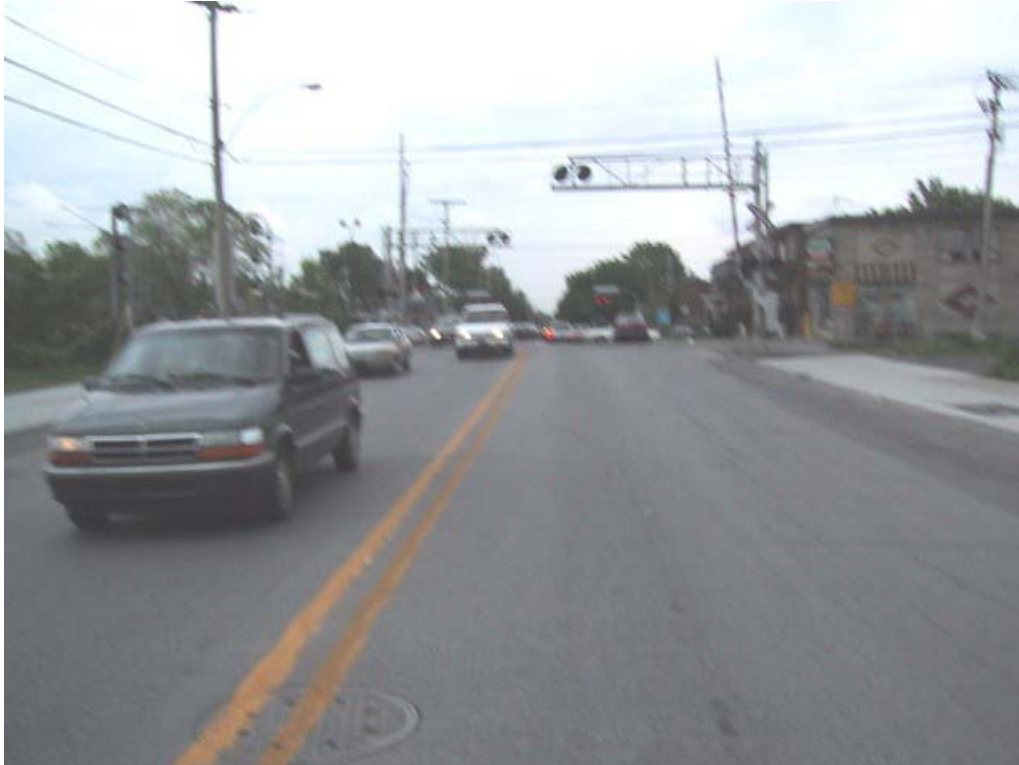
O'Brien Avenue – Southbound
