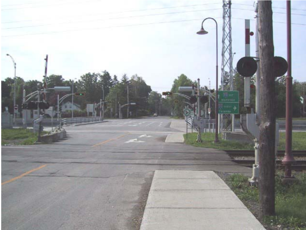
Woodland Avenue – Southbound West Sidewalk
