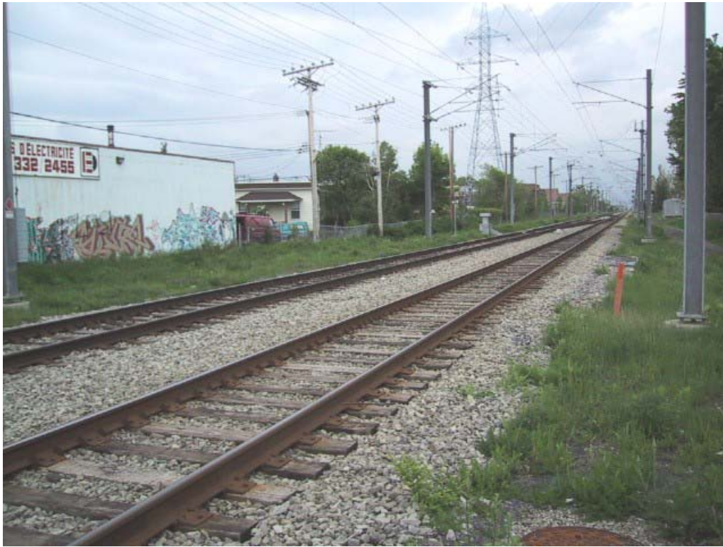
O'Brien Avenue – Southbound Looking West Along Tracks
