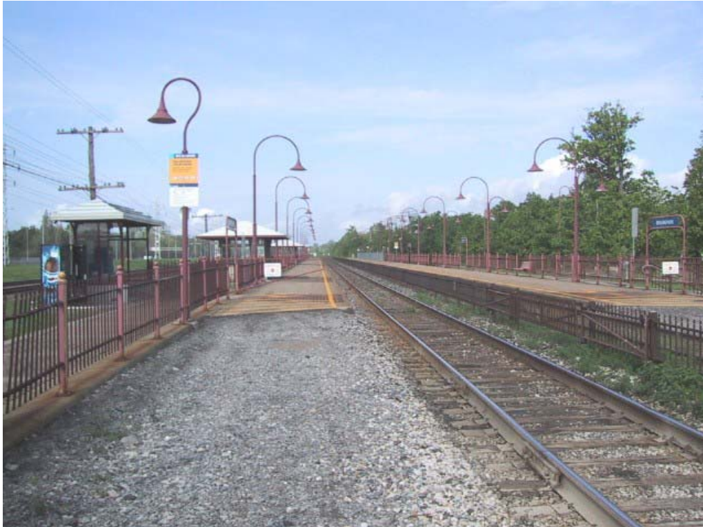
Woodland Avenue – Northbound Looking West
