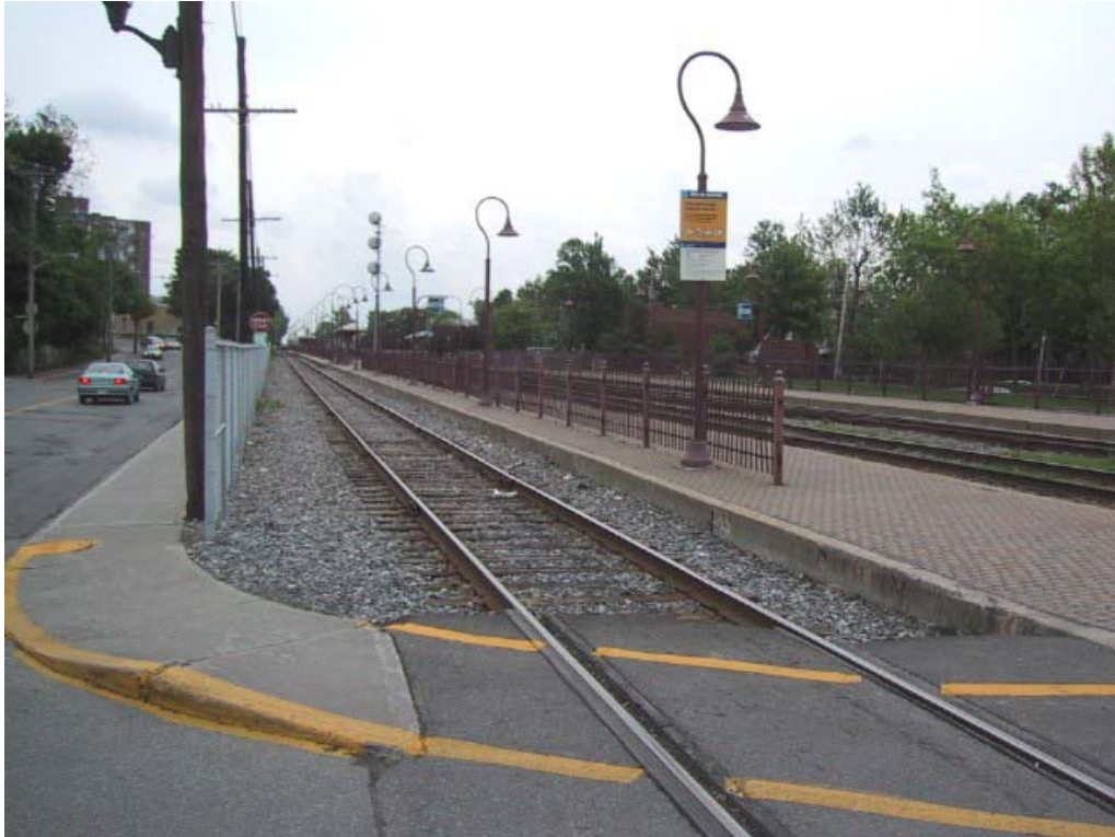
Westminster Avenue – Southbound Looking East Along Tracks
