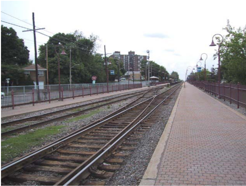
Westminster Avenue – Northbound Looking East Along Tracks
