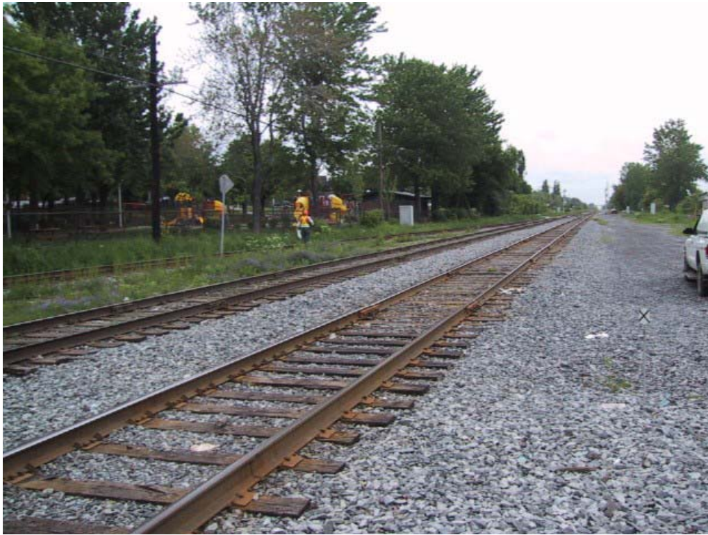
Elmhurst Street – Northbound Looking East Along Tracks
