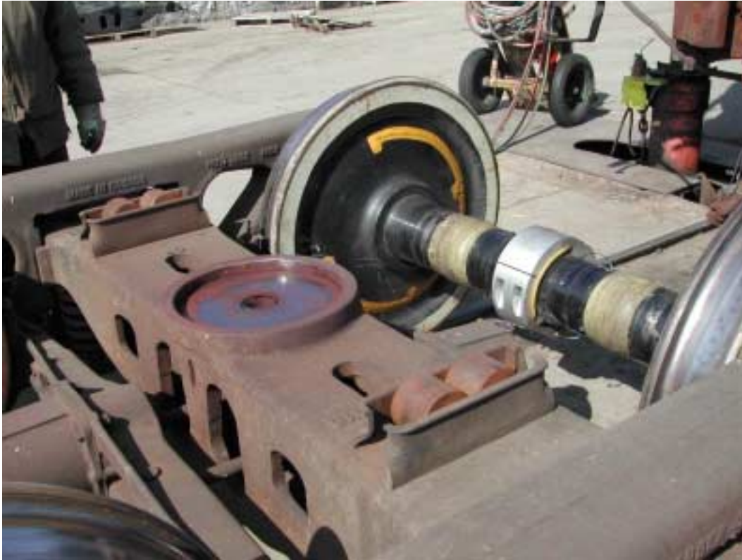
Figure 4 Instrumented wheelset during installation
