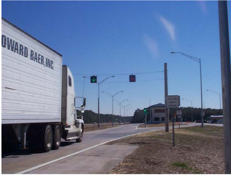
Figure 14. Typical Lane Control Signals (Red X Green Arrow)
