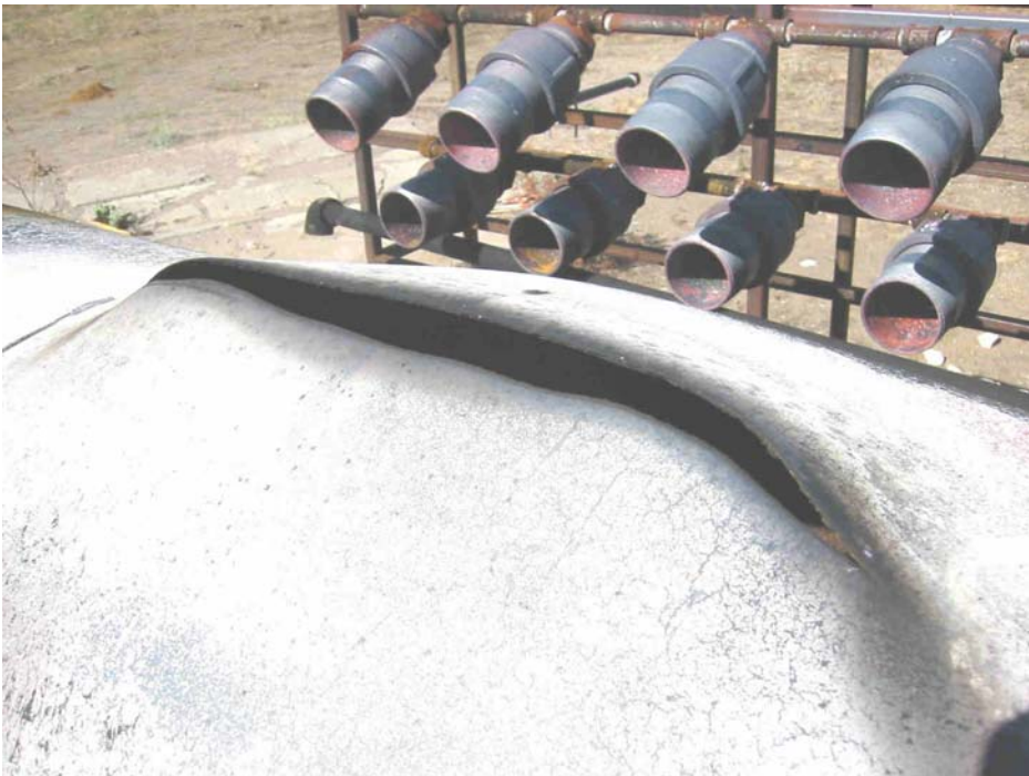
Figure 4.13: Tank failure, Test 04-6
