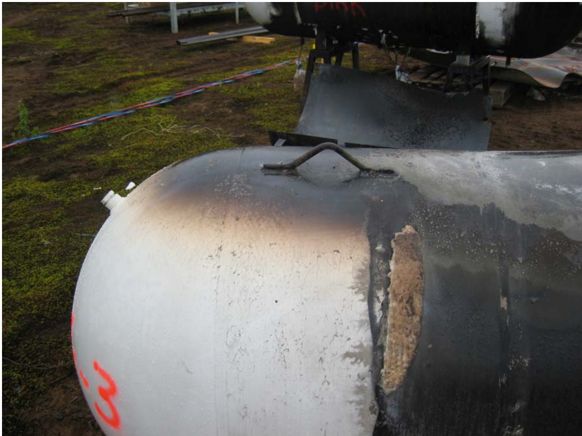
Figure 4.29: Test 04-03 burned vapour space wall under insulated area (not under fire)
