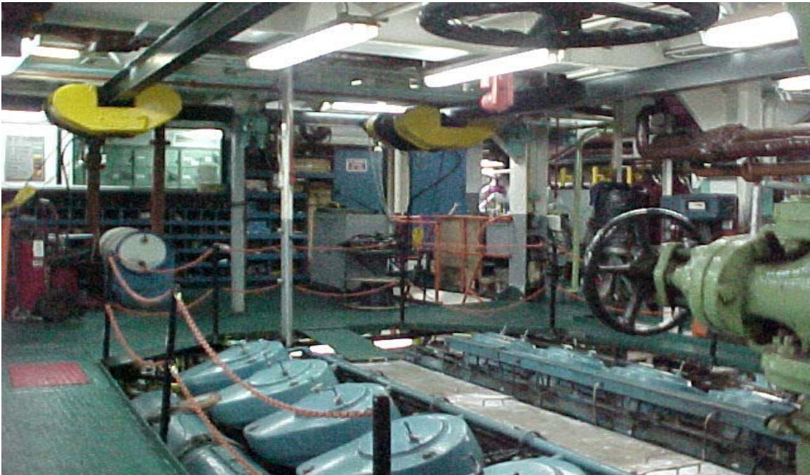
M.V. Cabot Engine Room (upper level, aft port)
