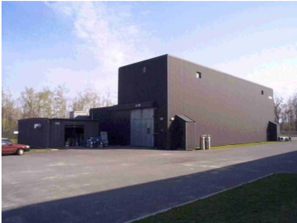
Photo 3.4: Exterior View of the NRC Facility
