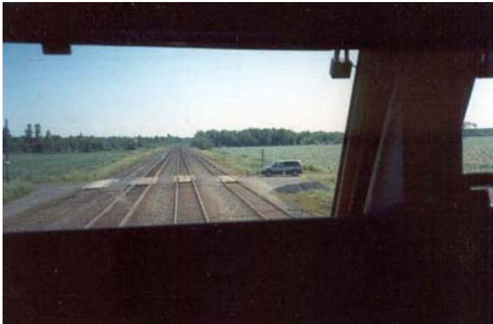
Figure 8: Private crossing – typically for farmers – without active warning systems
