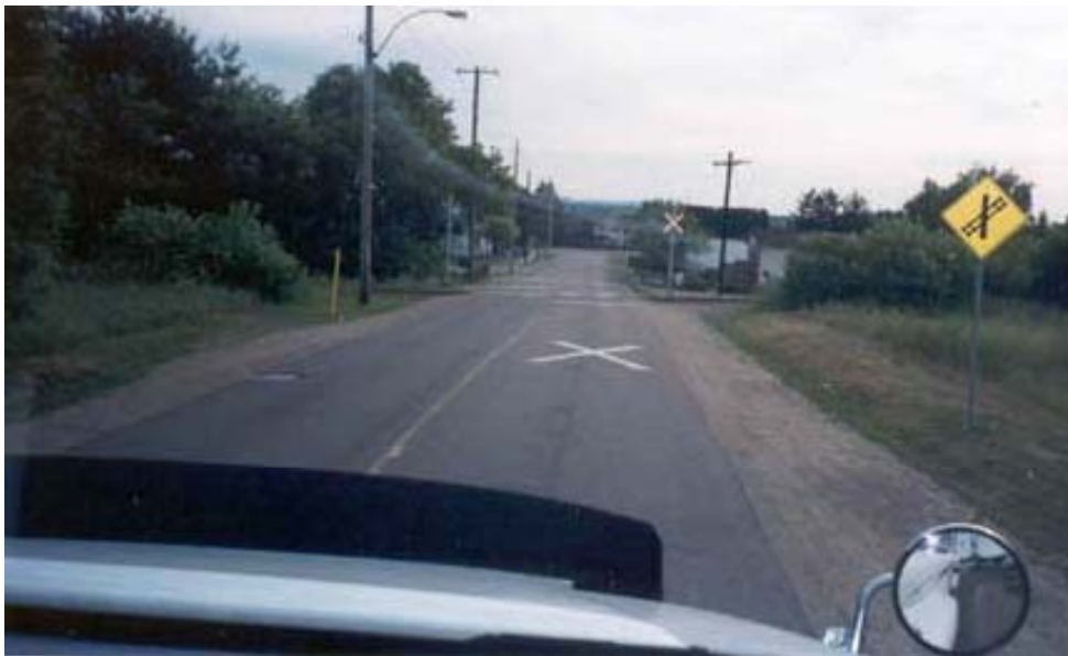
Figure 4: Vehicle approaching active crossing in Ontario with warning sign at right, pavement marking "X", and crossbuck with lights
