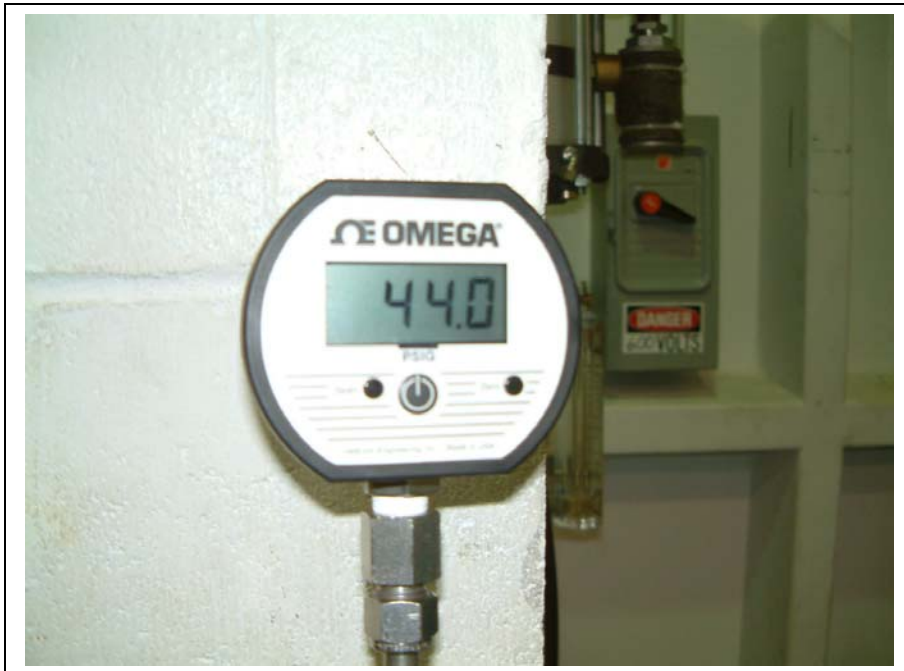
Photo 14 Drum Set C: Pressure test - Maximum pressure reached, no leaks
