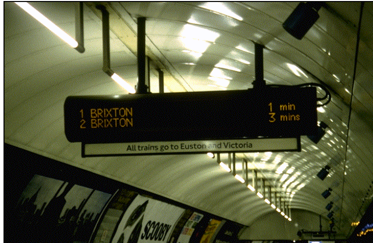
Figure 8a Display of the waiting time and destination of the next two trains from an underground (subway) station in London
