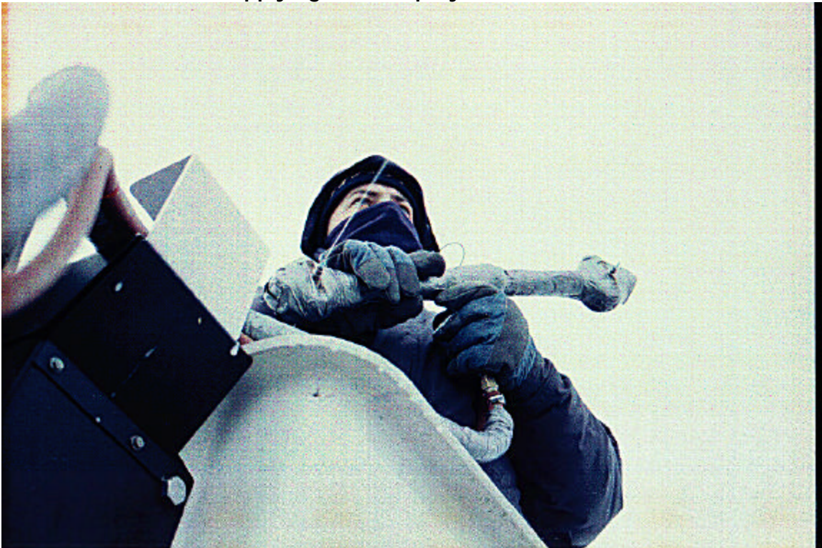
Photo 2.8 Applying Water Spray from Bucket
