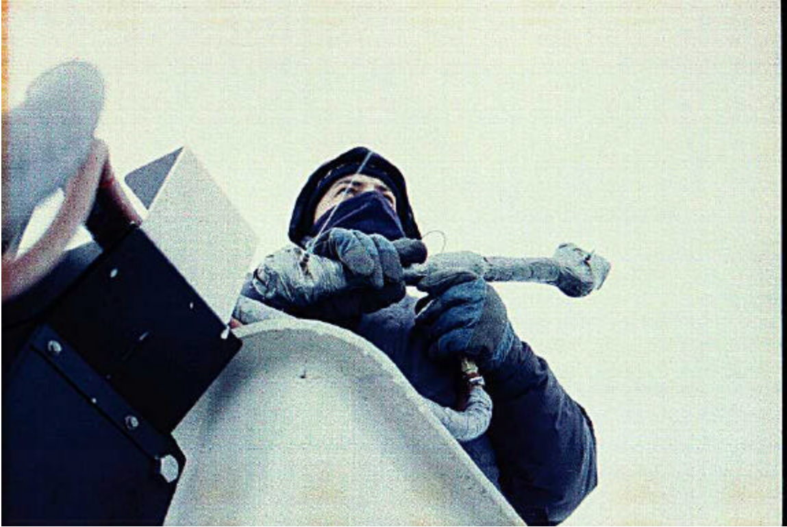
Photo 2.11 Applying Water Spray from Bucket
