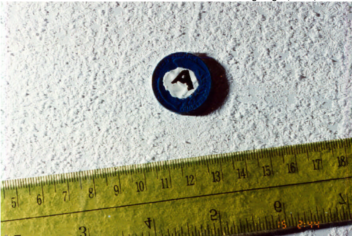
Photo 4.20 Plan Photo of the Frost Formation on the Trailing Edge (ID# 3)
