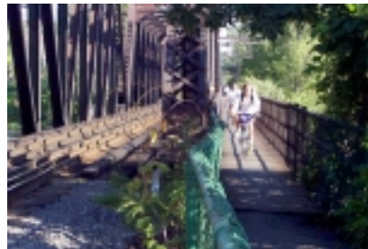
Bike-foot path alongside a railway bridge
