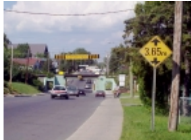
Advance clearance height sign
