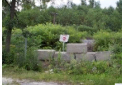
Fence needs to be extended
